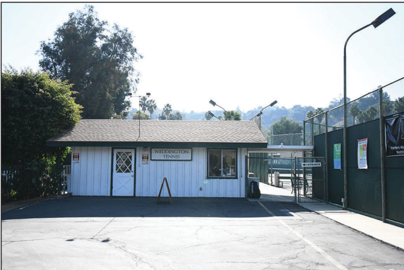
PHOTOGRAPH 3: Existing tennis check-in building. Tennis court fencing is visible in the right of the photograph.
