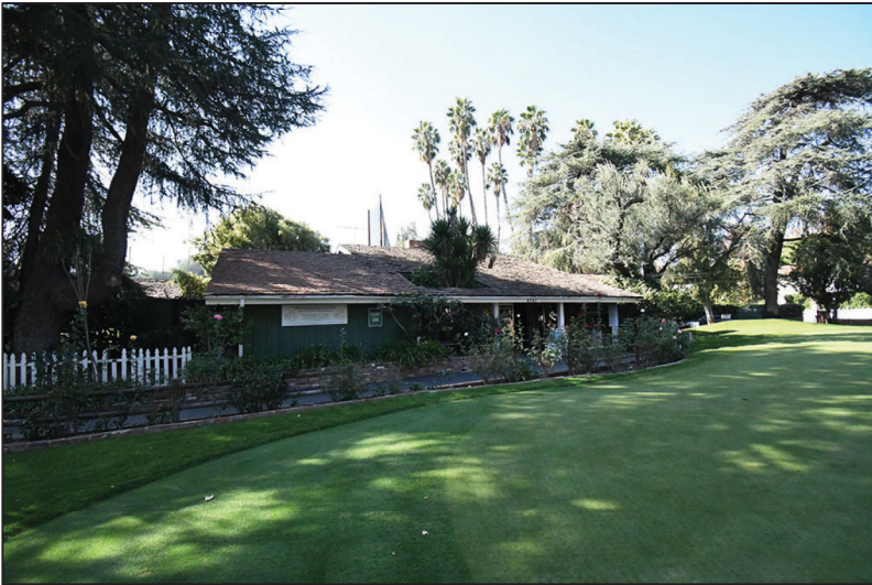
PHOTOGRAPH 1: The existing Weddington Golf & Tennis Clubhouse, which will remain as part of the River Park Project.
